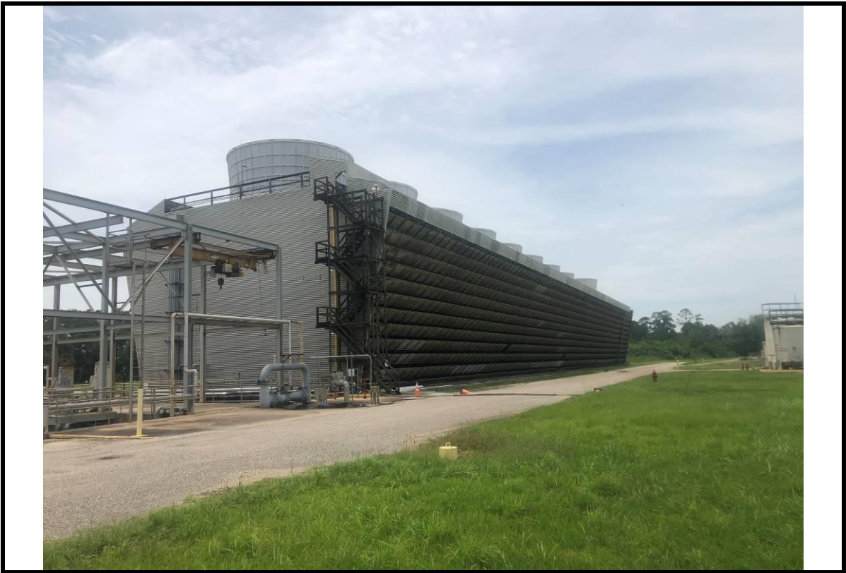
Photo 3: Unit 5 Cooling Tower, facing northwest.
