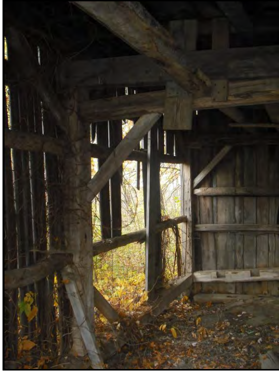
FIGURE 8. FEATURE 2 AT SITE 33LN0284; FACING SOUTHEAST
