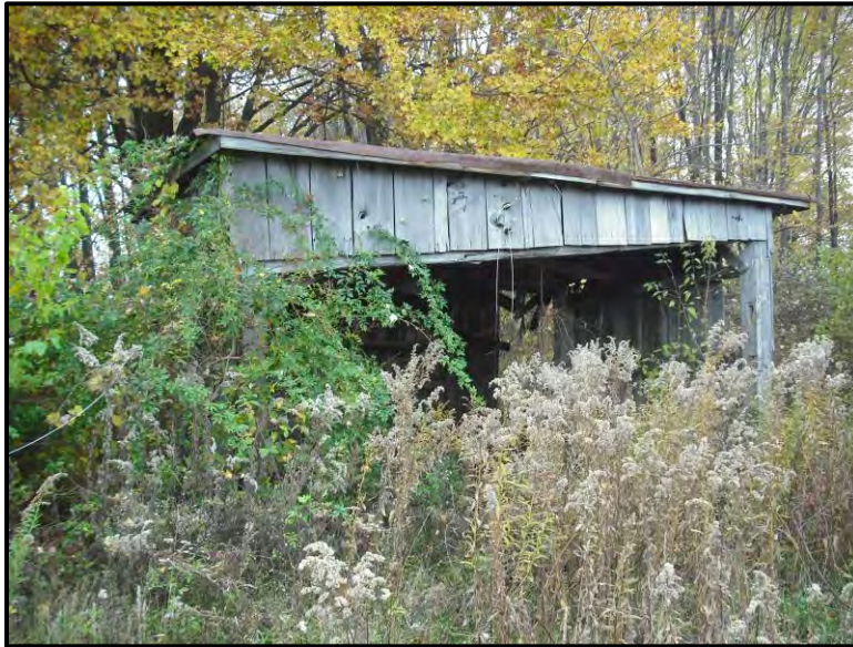
FIGURE 6. FEATURE 2 AT SITE 33LN0284; FACING SOUTHEAST
